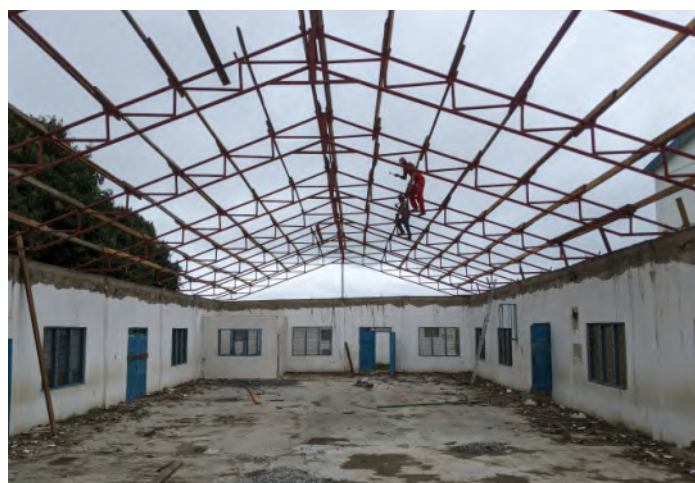
Metal trusses being erected on the Gaylon and Deanna Smith Hall
